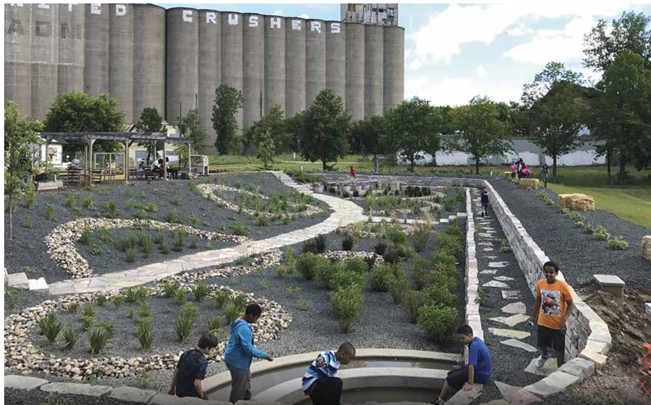
Towerside District Stormwater Management System
