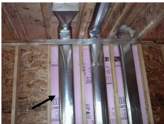
-1 1/2 rigid foam insulation used behind heat runs in exterior walls.
