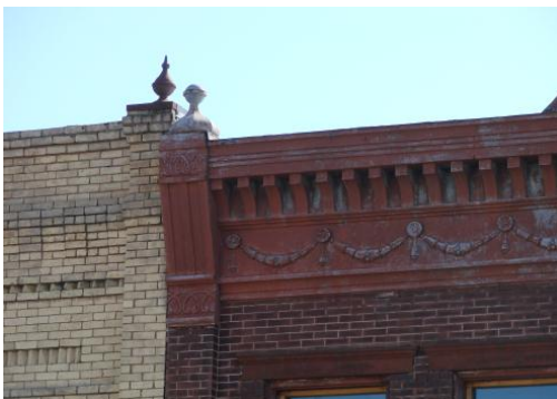
Cornices of the Corner Bar and Rynda Hardware buildings
