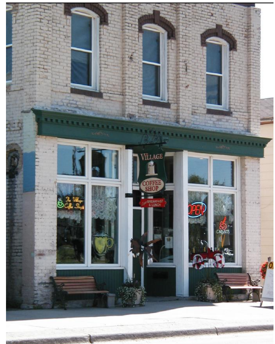
These renovated windows in the former West End bowling alley show how opening up windows brings an older building back to life. The above picture shows the building prior to the renovation which restored the front windows in 2002.
