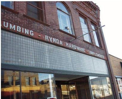
The Rynda Building has a wonderful transom window. These were very useful in a time before electric lighting
