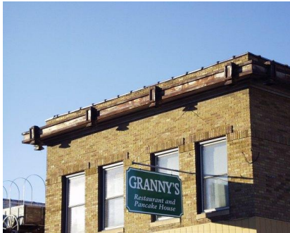
Renovating and maintaining cornices, like this one above Granny's restaurant, might seem an expense for no commercial gain and removing it is tempting, but how does that affect the charm of the stripped building? And what effects will that in turn have on business?
