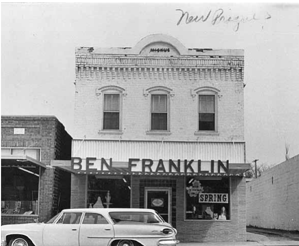
This building has been demolished and replaced with a parking lot.
