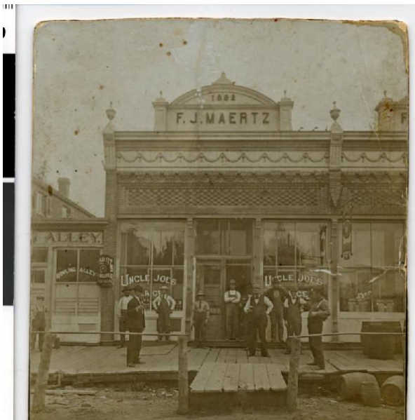
This building once stood where West End Liquor now stands, on the west end of the historic Main Street.
