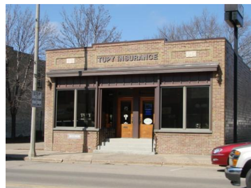
Beautifully restored windows, surrounded by copper.
